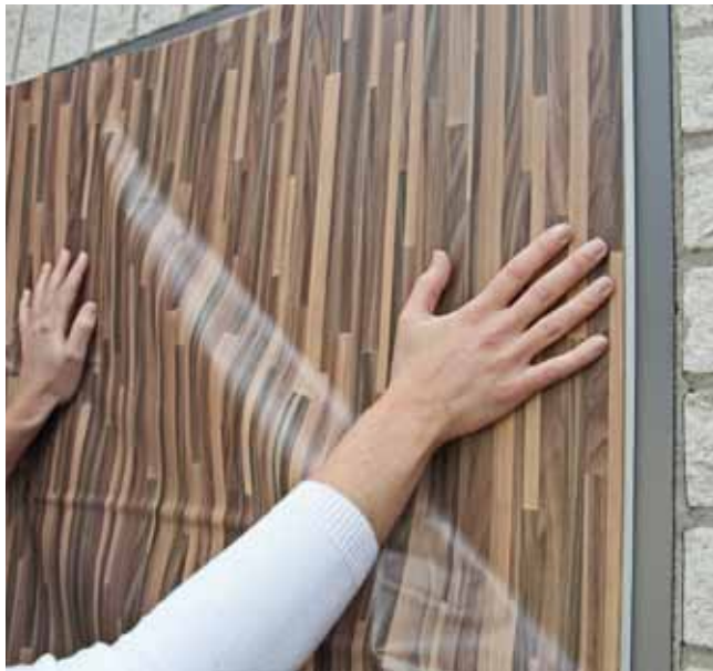
Apply foil, starting from one corner.
