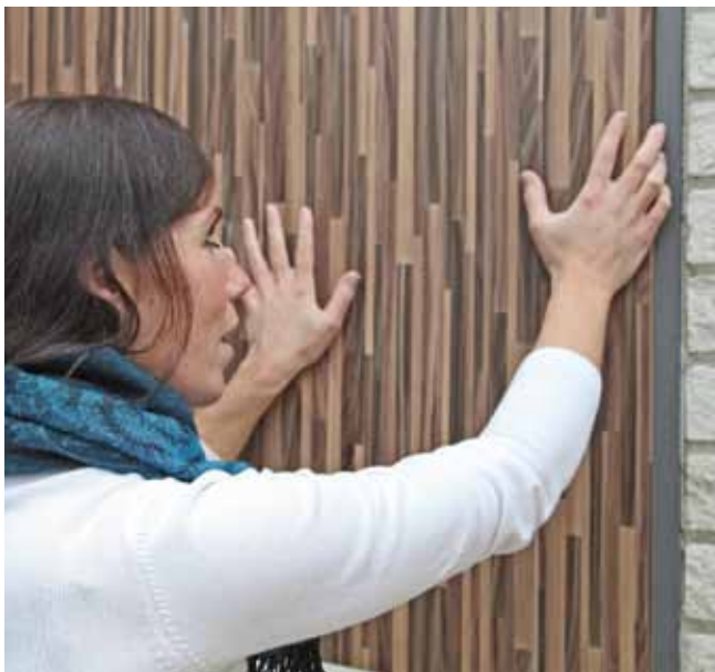
Remove backing and simultaneously smooth out foil.
