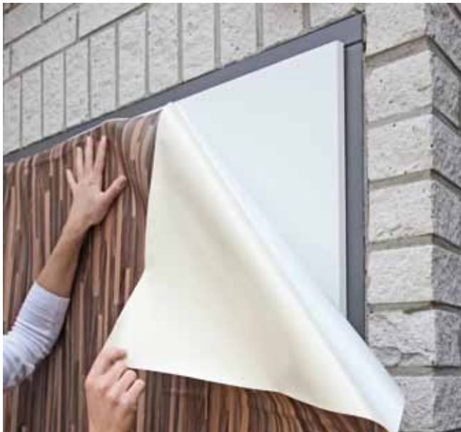
Cut foil to size and remove paper from foil.
